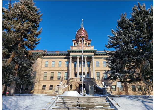
SOUTH ELEVATION - ORIGINAL ENTRANCE
