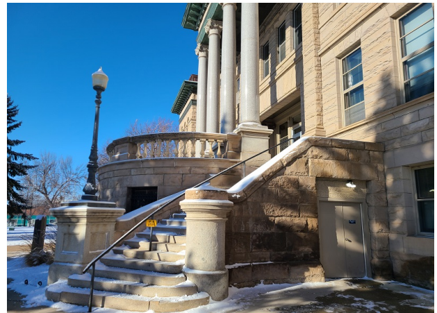
ORIGINAL / MAIN ENTRANCE / PORTE COCHERE
